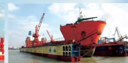
5万吨级“长山”坞 50,000 DWT Floating Dock: "Chang Shan"
