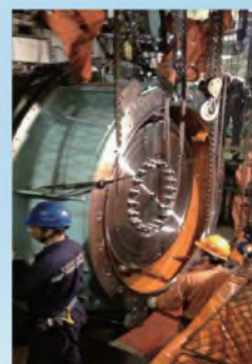
减震器拆解检修 Damper overhaul
