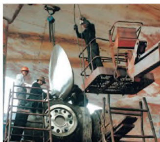
拆卸可变螺旋桨 CPP Dismantling
