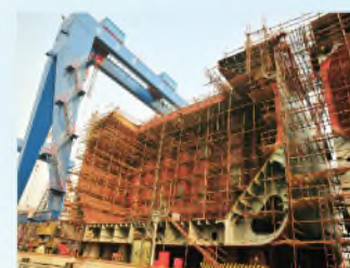
船舶分段中组建造场地 Block Assembling Site for Vessels.
