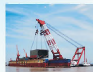
采用浮船坞合拢工艺建造灵便型船舶 Building handymax vessels by assembling the mega blocks in the floating dock.
