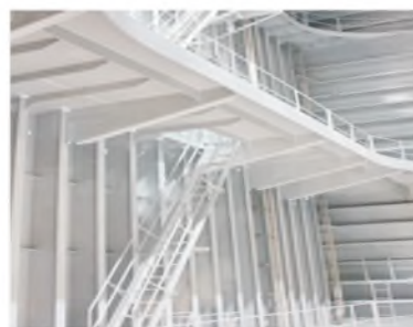
化学品船货油舱特涂 Apply of Interline 9001 in cargo tanks
