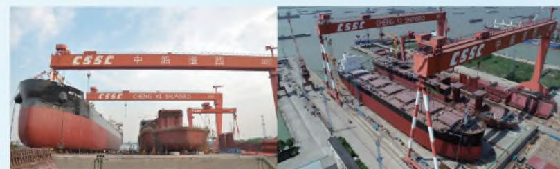
扬州公司10万吨级船台 The 100,000DWT slipway in Chengxi (Yangzhou)
