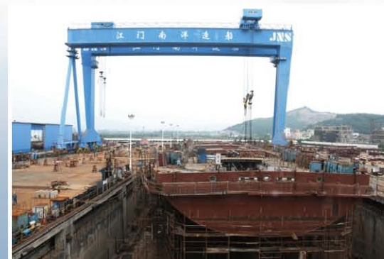
■ 船坞, 2台300吨龙门吊 (南洋厂区) Dry dock, 300t gantry crane x 2sets ( Nanyang Factory )
