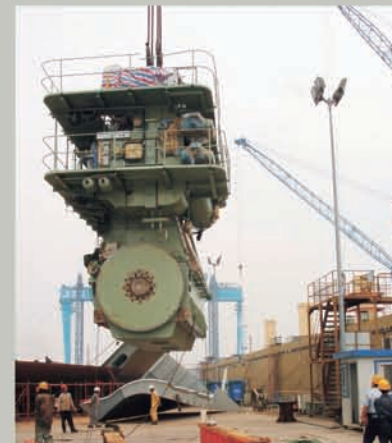
吊装主机 Main engine hoisting
